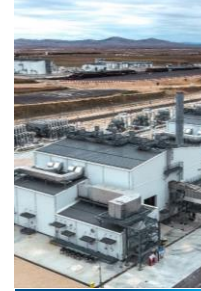
Gas Compressor & Metering Stations
